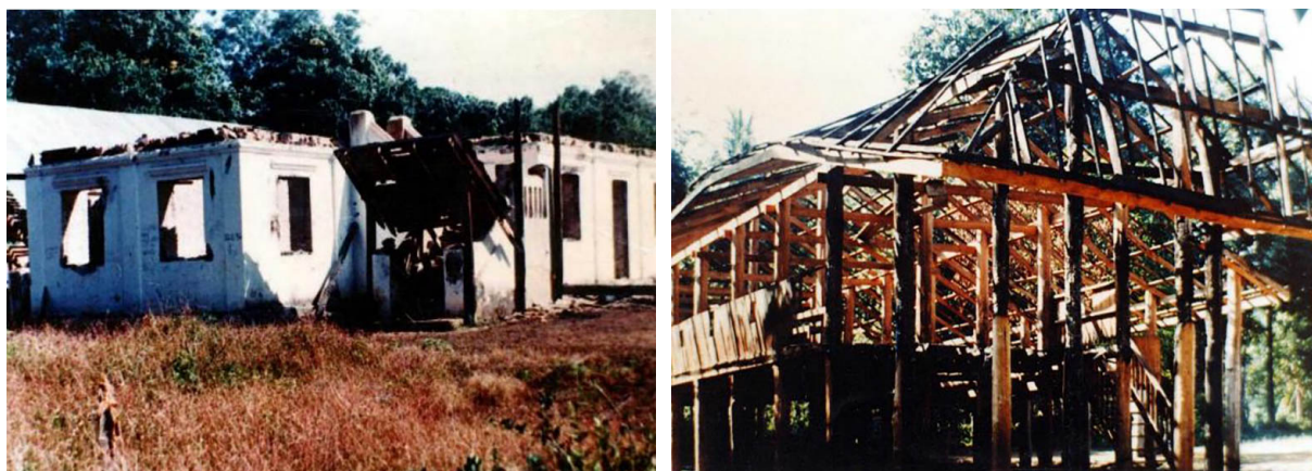
The church (on the left) and middle school (on the right) in Htee Ghuh Thaw village tract, Kruh Tu Township, Dooplaya District, burned and destroyed by SLORC troops of LIB #546 (under Major Tin Aye) and DKBA troops (under Pa Day) on November 22nd 1996 for no apparent reason other than to show the villagers who is in control. The troops also beat up the church pastor and burned down his house. [Photos: KORD]
