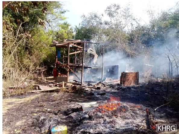
This photo was taken in February 2024 in Wr--- village, Hkay Kyi village tract, Moo Township, Kler Lwee Htoo District. On February 17 th 2024, at around 11 am, SAC LIB #439 conducted a drone attack in Wr--- village by dropping bombs. The photo shows a house that was burned by the air strike. [Photo: KHRG]
