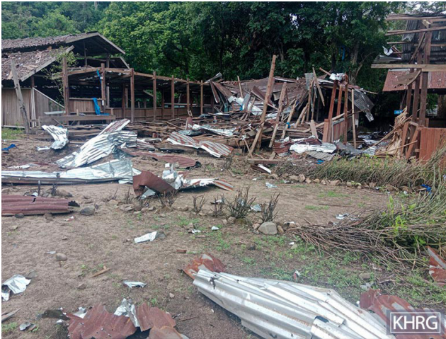
This photo was taken on July 21st 2023 in Pay Kay village tract, Lu Thaw Township, Mu Traw District. This photo shows Cf--- school buildings destroyed by an SAC air strike on June 27 th 2023, when an SAC fighter jet dropped two bombs on the school. [Photo: KHRG]
