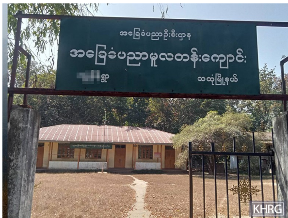
This photo was taken on January 10 th 2024 in I--- village, Kaw Ler village tract, Tha Htoo Township, Doo Tha Htoo District. It shows the I--- school (under Burma government administration), empty of students and teachers. The school buildings were partially damaged by shrapnel from SAC shelling in December 2023. [Photo: KHRG]
