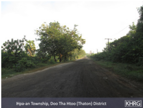
This photo was taken on October 31 st 2019. It shows the road that goes to the Myaing Ka Lay cement factory. Its colour is turning into black or dark blue because of the coal dust that falls when coal is being transported to the factory. [Photo: KHRG]
