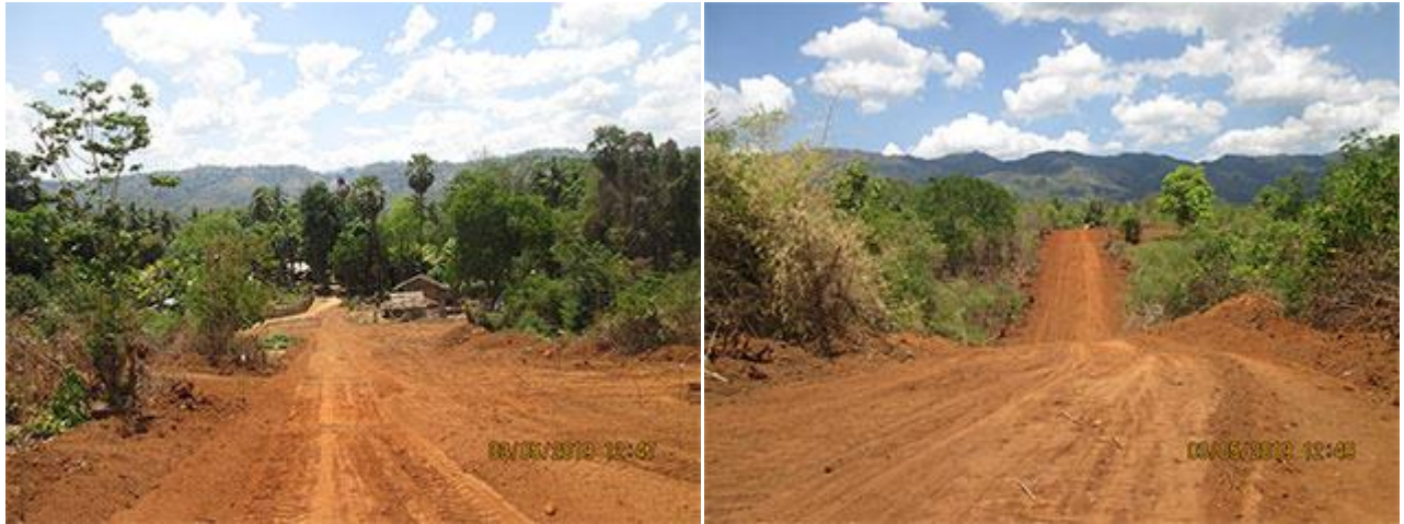
These two photos were taken on May 3 rd , 2019 in L--- village, Meh Klaw village tract, Bu Tho Township, Hpapun District. These two photos show the road that was constructed in K---.
