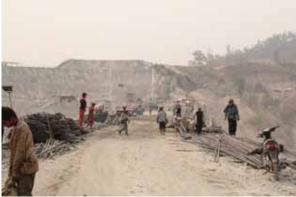
The photos above were taken in March 2012 in the Day Loh River Valley. The top two photos show construction workers building cement terraces, reinforced with bamboo poles, which together will contain the water once the dam becomes operational. In the background, features characteristic of excavation for unknown purposes are present. [Photo: KHRG]
