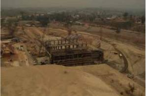
The photos above show two different views of the powerhouse that will produce electricity from the dam. The yellow pipe beneath the powerhouse allows water to enter and connect to the machine that produces hydropower. [Photos: KHRG]
