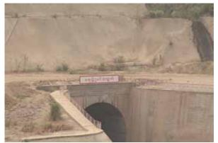
The photos above show electricity pylons on a different side view of the Toh Boh Dam under construction. In the photo above right, the sign in red reads: "*Tunnel for diverting water out*." <sup>4</sup>[*Photos: KHRG*]
