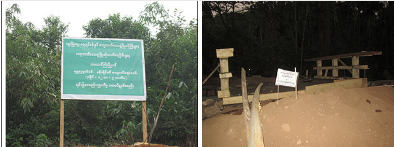
The first photo shows a signboard regarding road construction that was erected by Chan Mya Way Si Company, in Thandaunggyi Township, Toungoo District, taken on July 11 th 2015. The signboard reads that the company is constructing the road between T--- and S--- villages. The second photo was taken on July 6 th 2015 between T--- and H--- villages, Thandaunggyi Township. The photo shows one of the bridges and roads that were constructed by La Thitsa Pan Ka Maing Nin Company in the summer of 2015. [Photos: KHRG]
